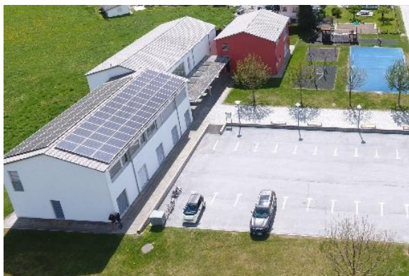
PV-Anlage MZH in Agarn
